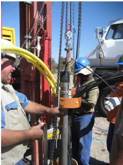
**Figure 2.7 - Assembly of sub-electrode element FOR Vertical Well type Electrode**
