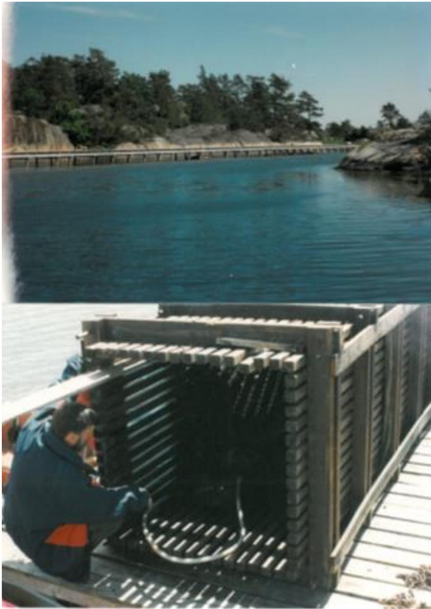
**Figure 2.13 - Sea Electrode Graphite Sub-electrode in Coke in Wooden Cage**
