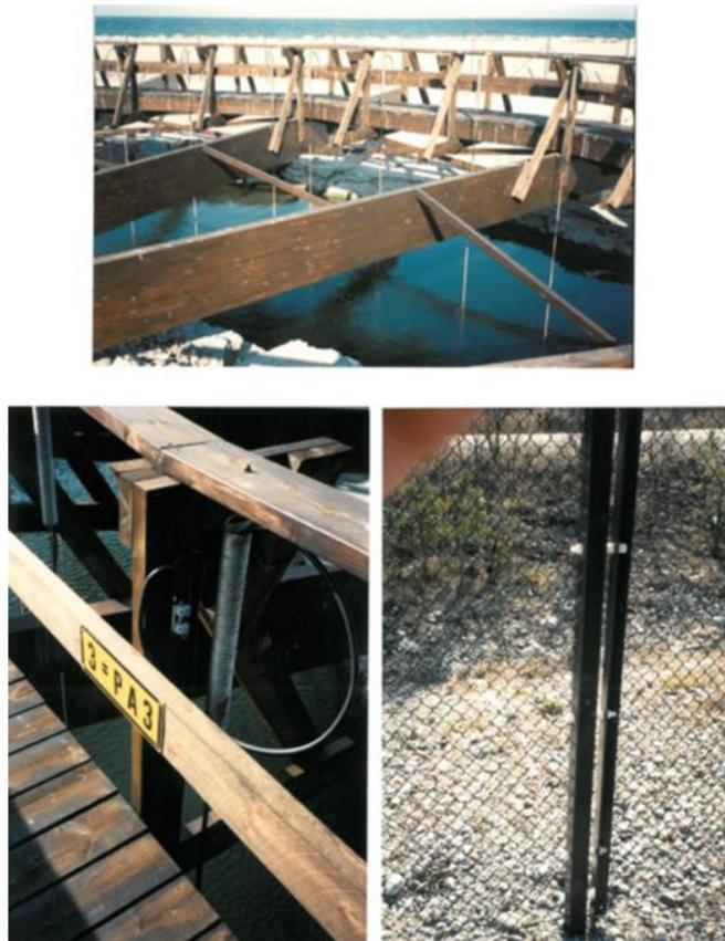
**Figure 2.17 - Pond Electrode with Sub-Electrodes Placed Directly in Seawater with Wooden Fence to Avoid Transfer Potentials**
