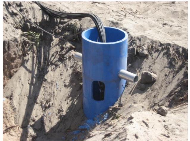
**Figure 2.8 - Completed sub-electrode assembly before inserting Vent pipe and filling with coke**
