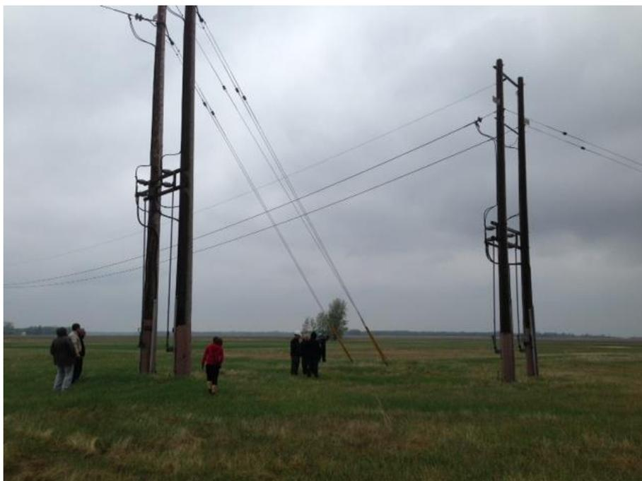
**Figure 7.4 - Electrode Site without Fence and Electrode Switches Mounted on Distribution poles**
