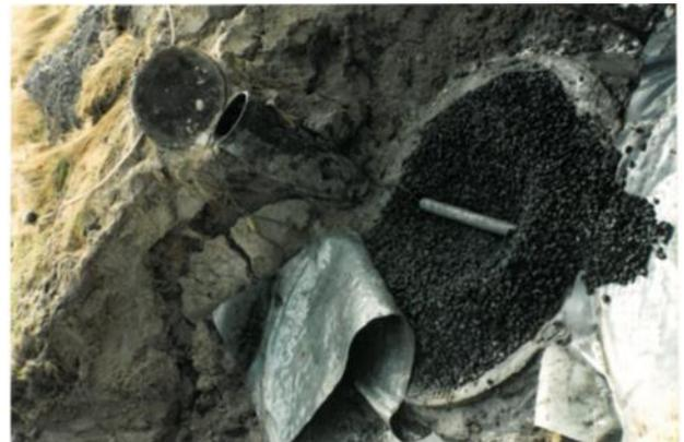
Figure 2.15 - Beach electrode in coke with covers to avoid Mixing of coke and soil
