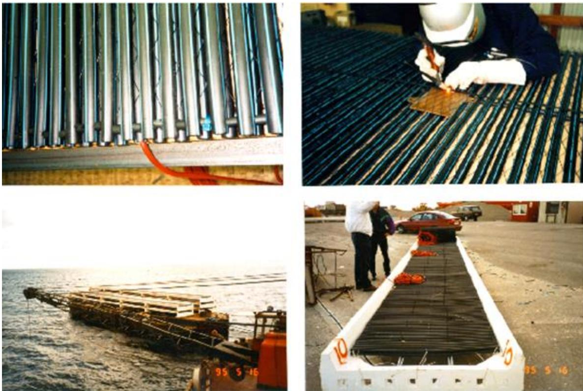
Figure 2.12 - Titanium Net Mounted in Concrete Frame
