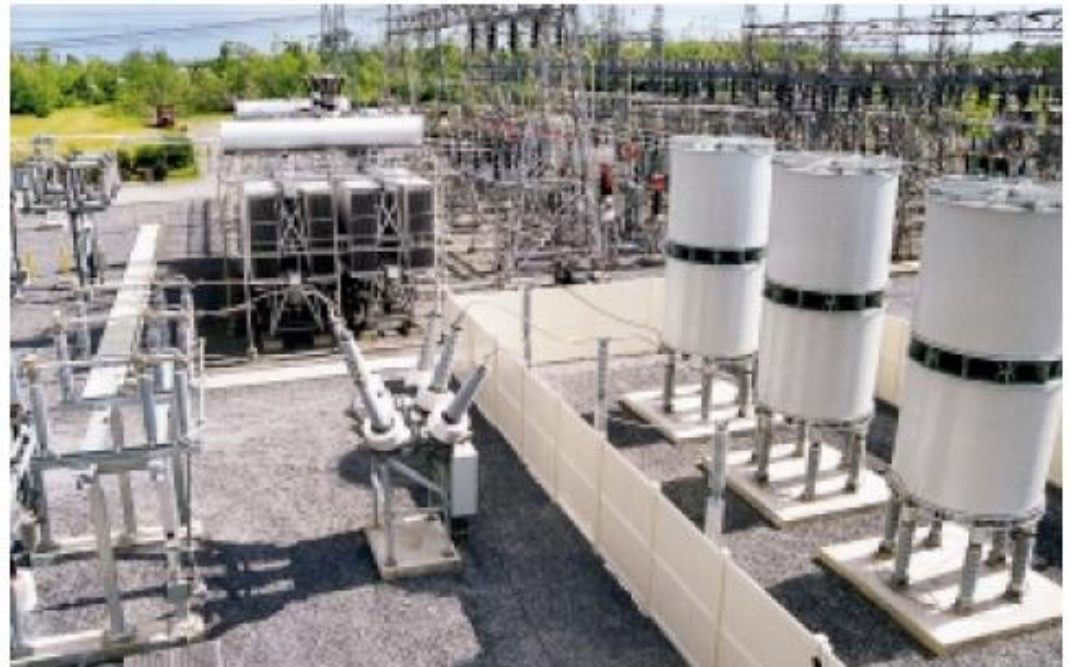
6 Plattsburgh APST, consisting of three single-phase inductors, a circuit-breaker, part of a disconnect switch, and the existing PST (at rear)
