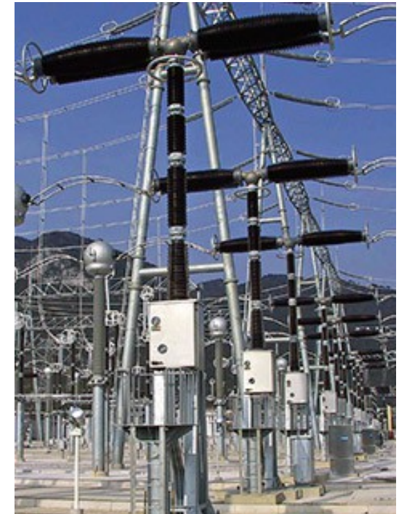
Live tank 550kV circuit-breaker
