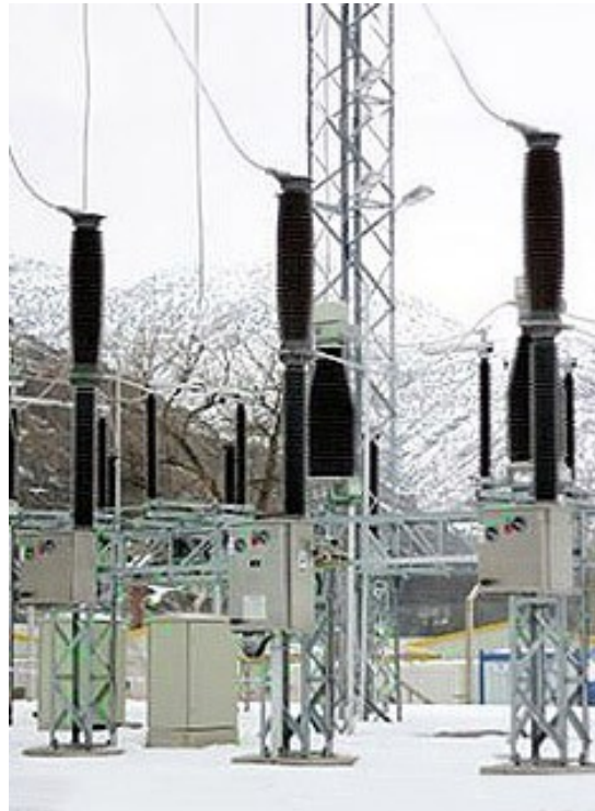
Live tank 245kV circuit-breaker
