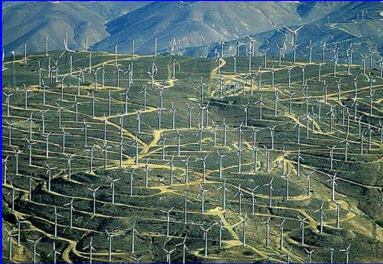
Tehachapi Pass Wind Farms
