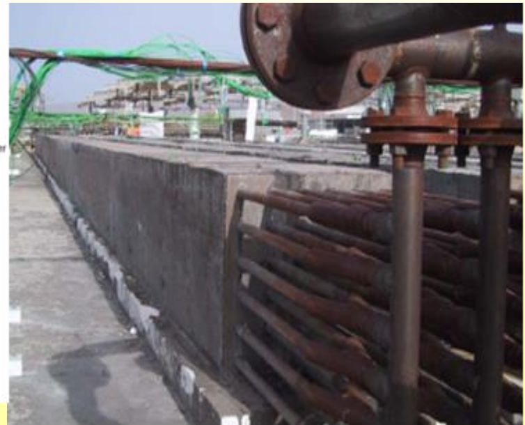
High temperature concrete storage system (Tamme 2003)
